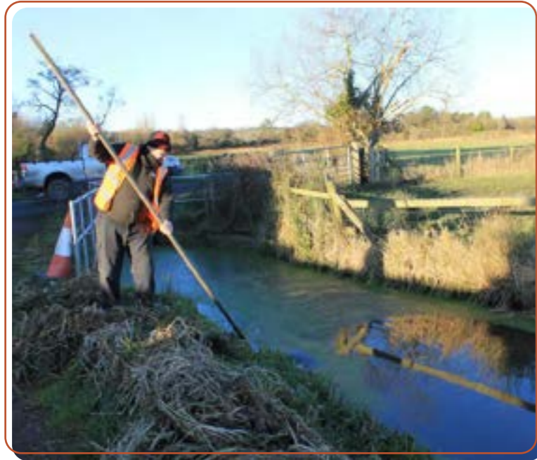
▲ Drashing: clearing vegetation in a reed using a longhandled hook © Gavin Jones/Living Levels Partnership
