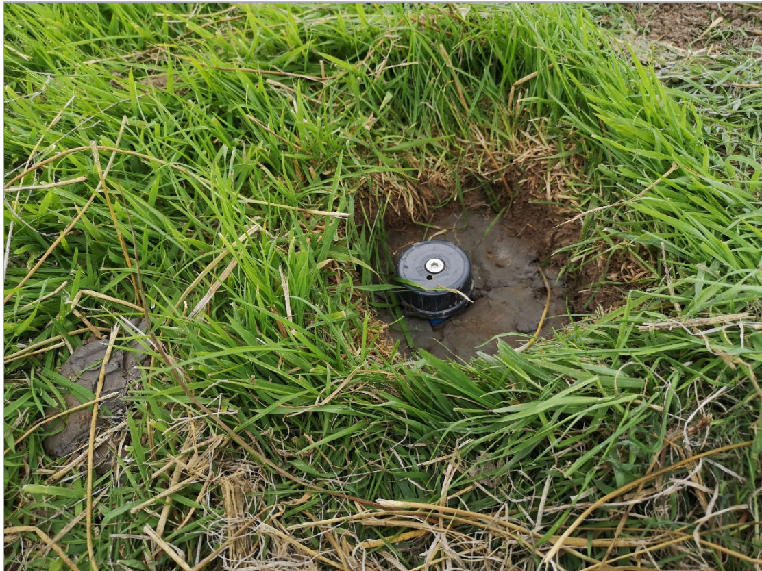
Figure 5.1-1. Dipwell (at Fair Orchard Farm) completed c. 30 mm below ground level to allow unencumbered farming operations.
