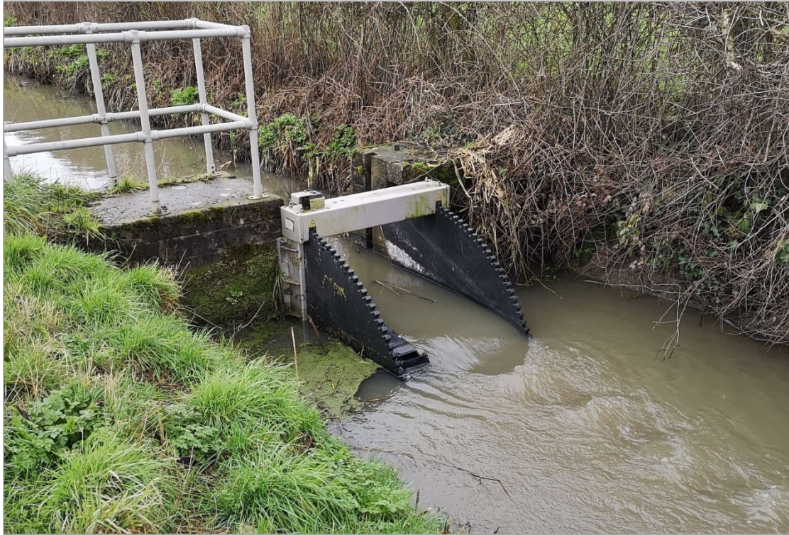
Figure 2.5-2. Sluice W11 on the Rhosog Fawr IDD reën, near to Sluice House Farm in the western part of the Wentlooge Level. The photograph was taken in January 2020, and the sluice is in its lower, colder month position, with flow towards the tidal gate c. 360 m downstream.
