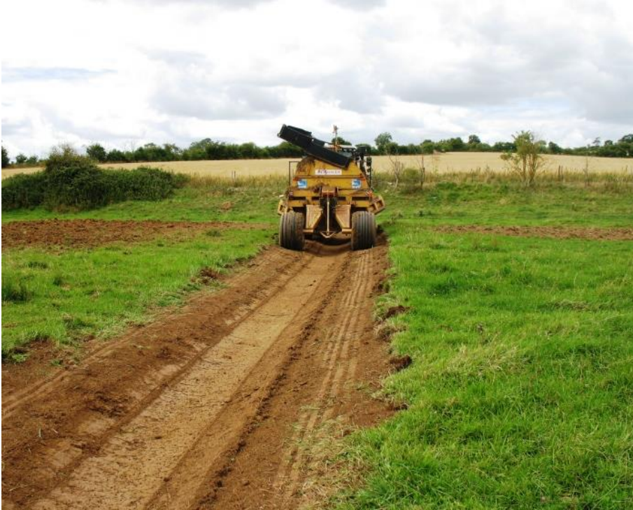
Fig. 3 - RSPB Rotary Drainer excavating a foot drain – the depth and width of the feature and spoil spreading can be adapted for use in the restoration of grips and furrows.
